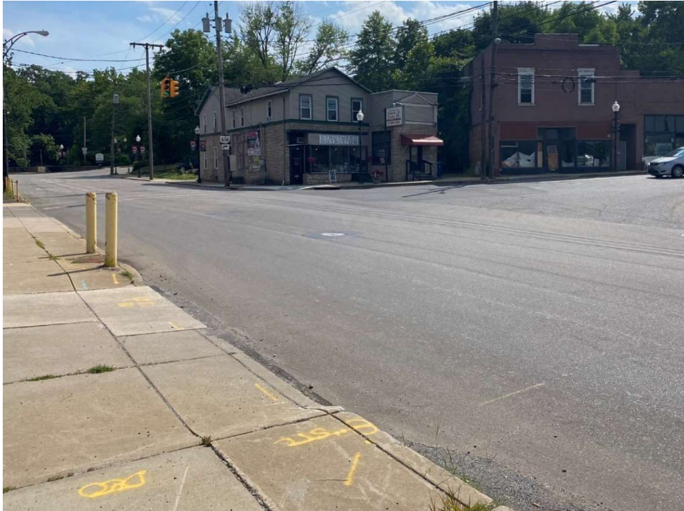
Figure 12 - Yellow bollards at catch basin inlet.
