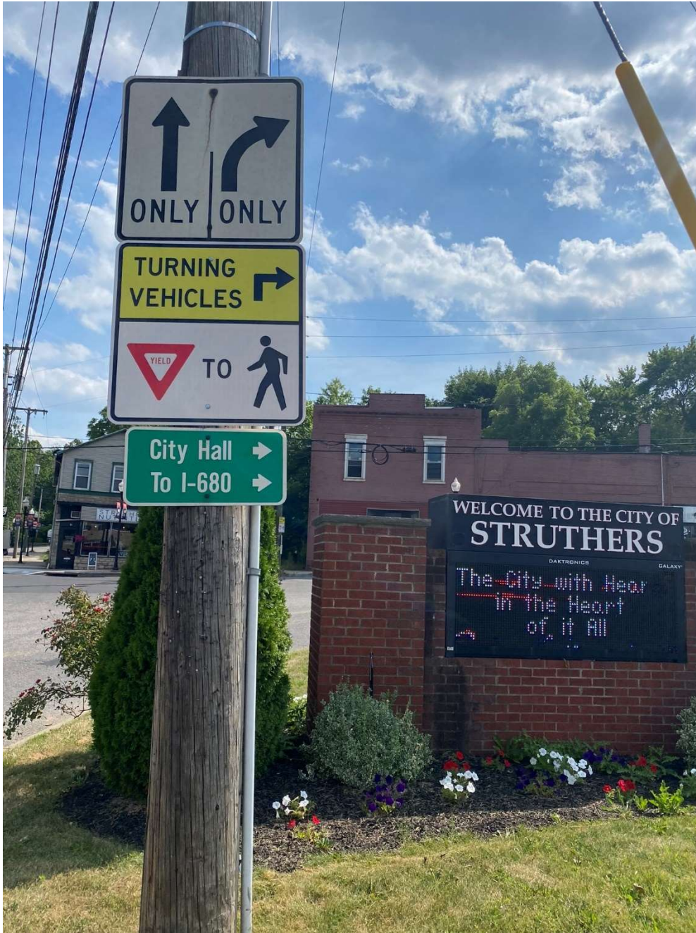
Figure 16 - R10-15 pedestrian crossing signage.
