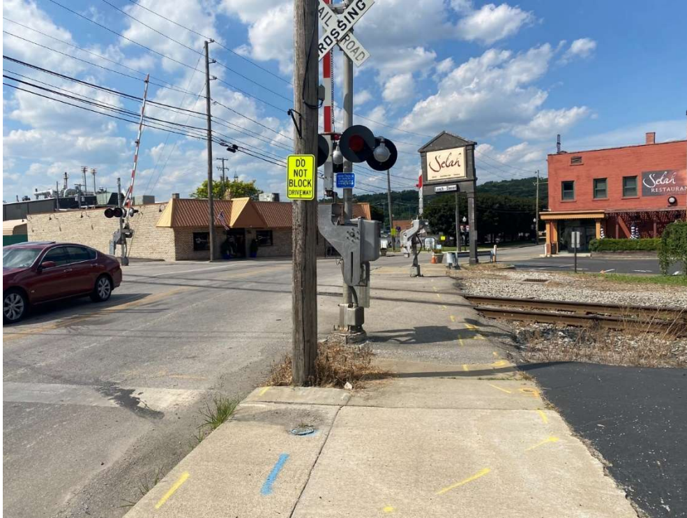
Figure 21 - Rail crossing with pedestrian and vehicular protection.
