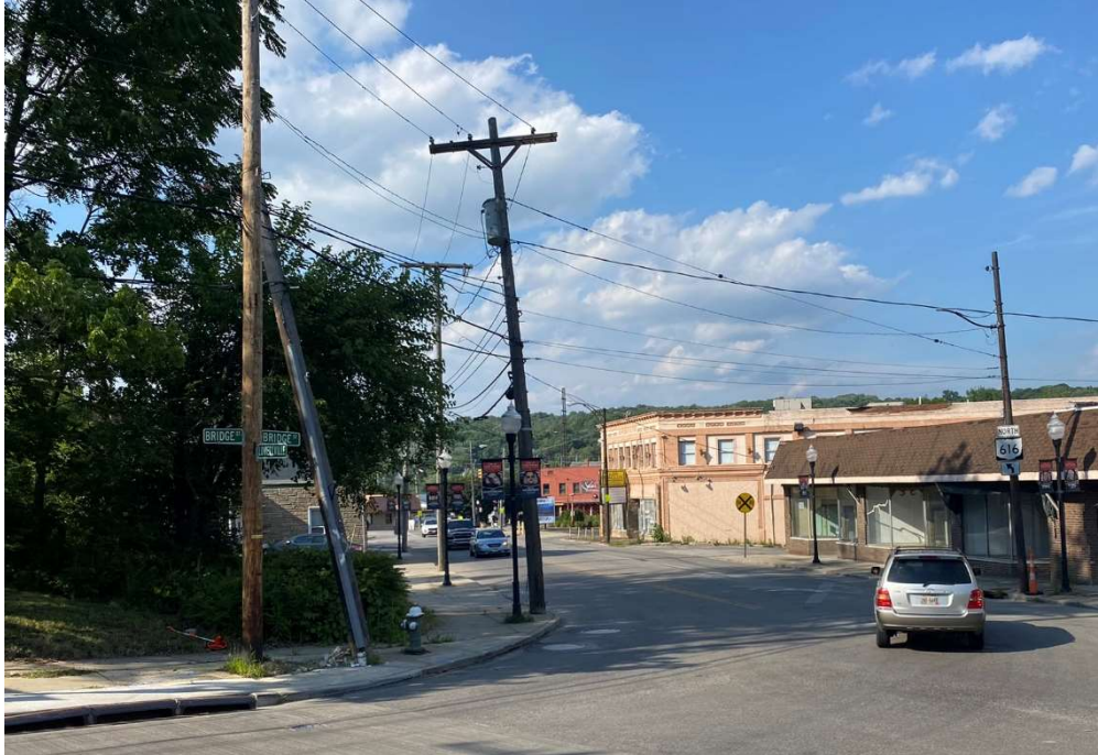
Figure 10 - Evident recent work with utility poles.
