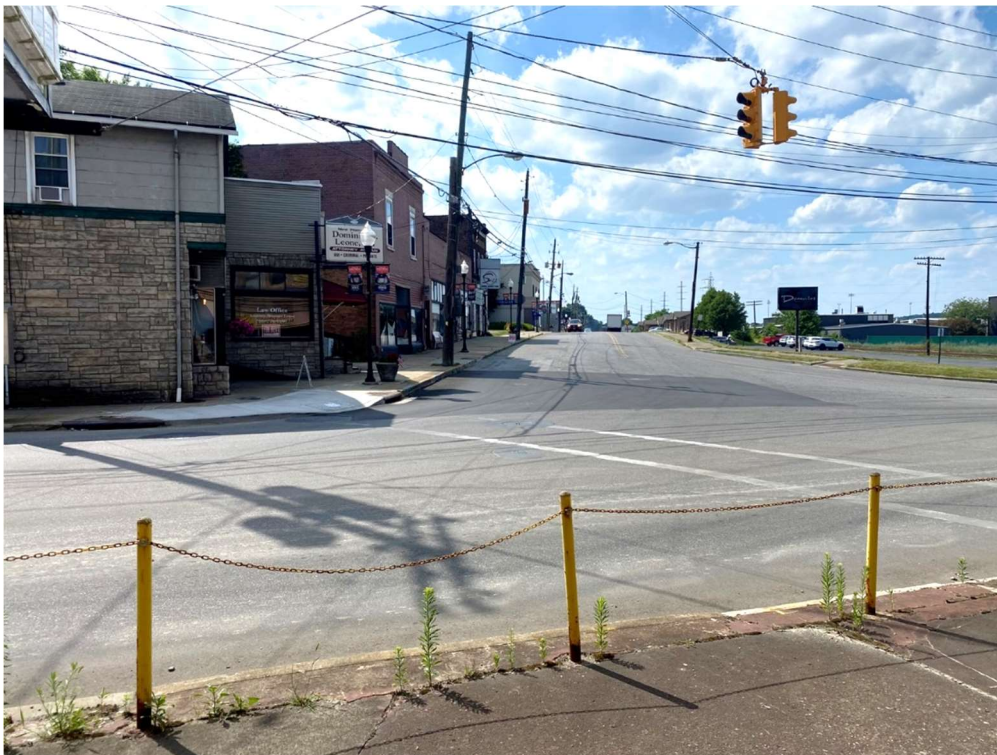
Figure 11 - Rusty chain rail directing pedestrians to driveway north of rail.
