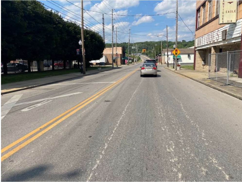
Figure 19 - View of Liberty Street intersection from South Bridge Street northbound.
