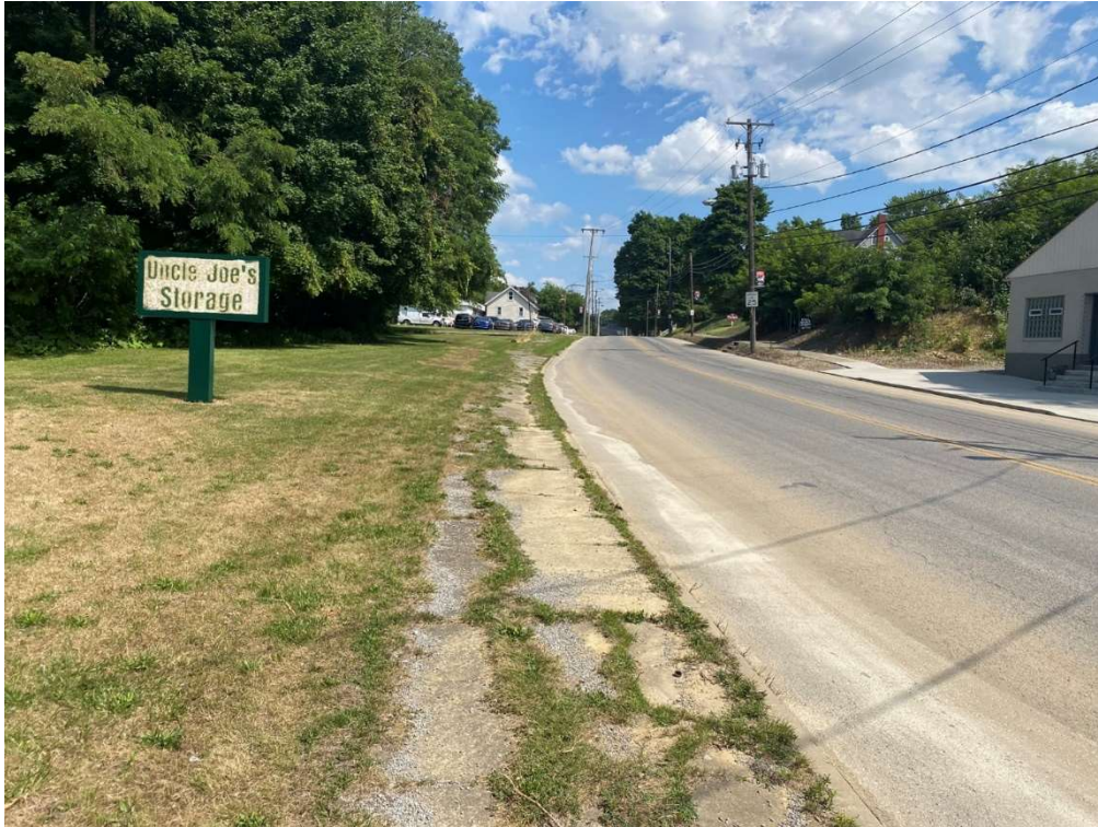
Figure 23 - Insufficient pedestrian facility south of South Bridge Street, east side of Lowellville Road.
