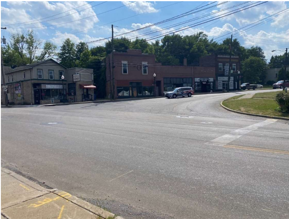
Figure 22 - Large curb return at State Street.
